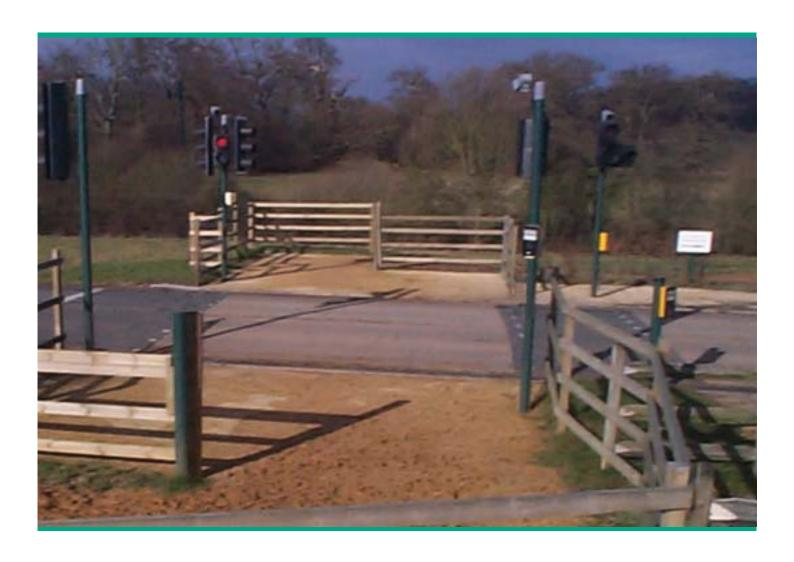
A minimum of 3 metres is needed between the two parts of the crossing to give adequate separation. The prescribed maximum is 5 metres in order to dissuade drivers from stopping between crossings, during the change from a vehicular green.
