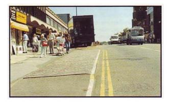
These can take a variety of forms, from large cobbles to brick on edge, as well as some specially designed types of paving. The paving will normally need to be at least a metre in width. It should not be laid where it would inconvenience or cause a danger to pedestrians, particularly disabled people and wheelchair users.
