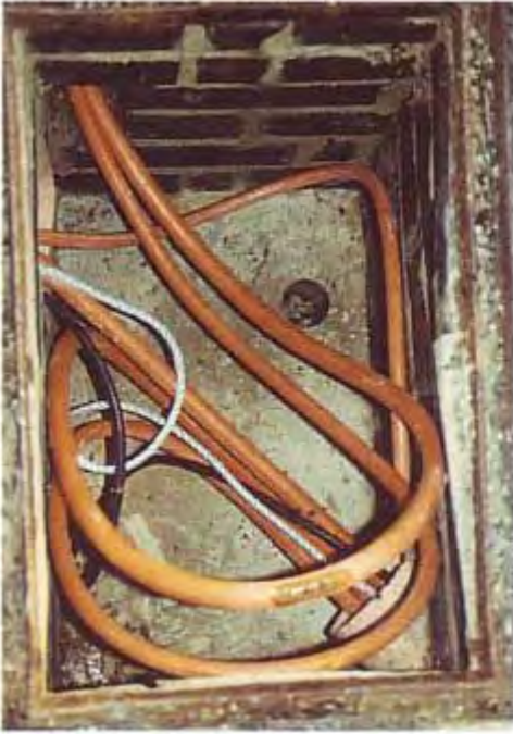
Drawpit showing traffic signal cables.
