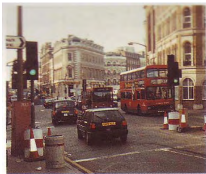
A typical temporary traffic signal set-up.
